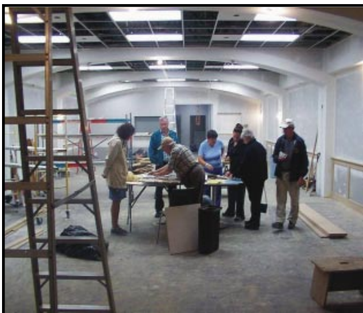
HALL RENOVATIONS UNDERWAY OCTOBER 2008
